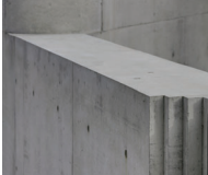
E - OFF-FORM CONCRETE CANDALEPAS ASSOCIATES - PERRY PARK
