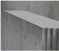
E - OFF-FORM CONCRETE CANDALEPAS ASSOCIATES - PERRY PARK
