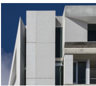
A - PRECAST CONCRETE CANDALEPAS ASSOCIATES - QT HOTEL PERTH
