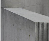
E - OFF-FORM CONCRETE CANDALEPAS ASSOCIATES - PERRY PARK
